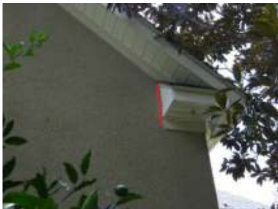
E. Seal roof terminations
