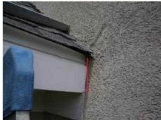
B. Insure soffit sealed to stucco
