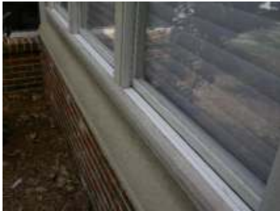
A. Seal all window perimeters
