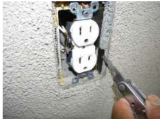
Misc- DEFS stucco applied over felt and OSB sheathing
